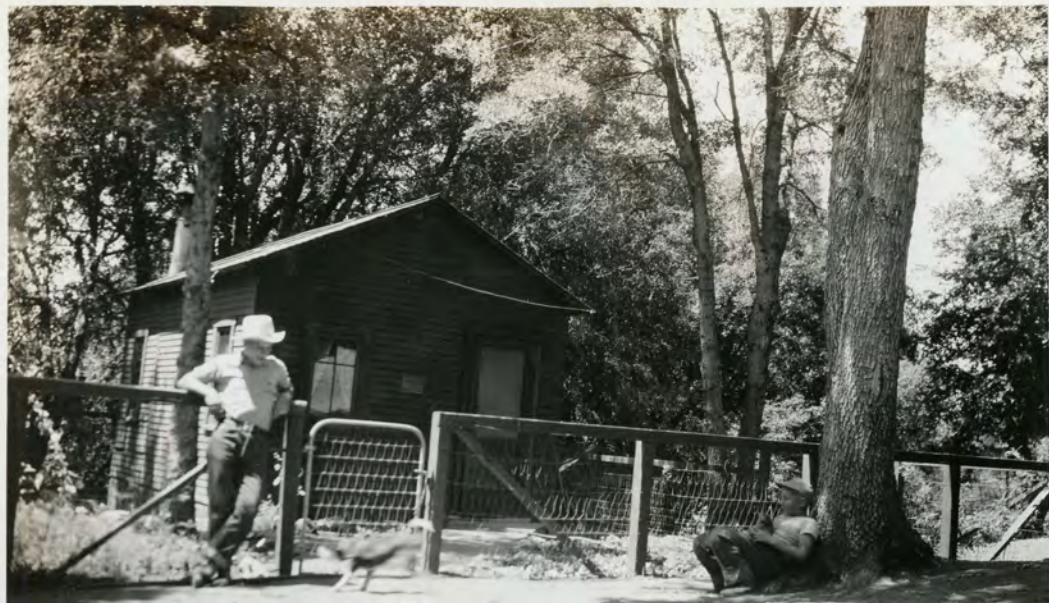
Skip + I at Chew's Ridge Guard Station
