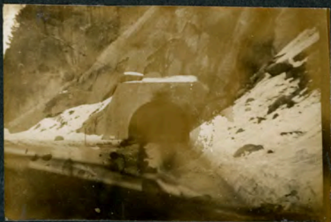
Tunnel on road to Badger Pass.
