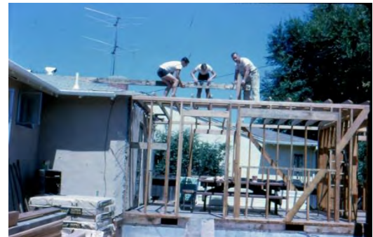
Getting the Framing up. Jim, Danny and me putting up the ridge pole for the roof and tying into existing house -- August 7, 1966
