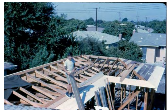
All Framing complete and starting on the roof sheeting. Handing boards up to Jim. August 27, 1966
