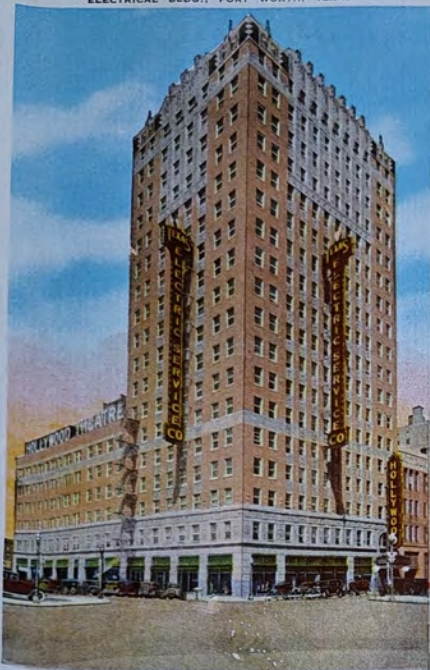
ELECTRICAL BLDG., FORT WORTH, TEXAS—9
