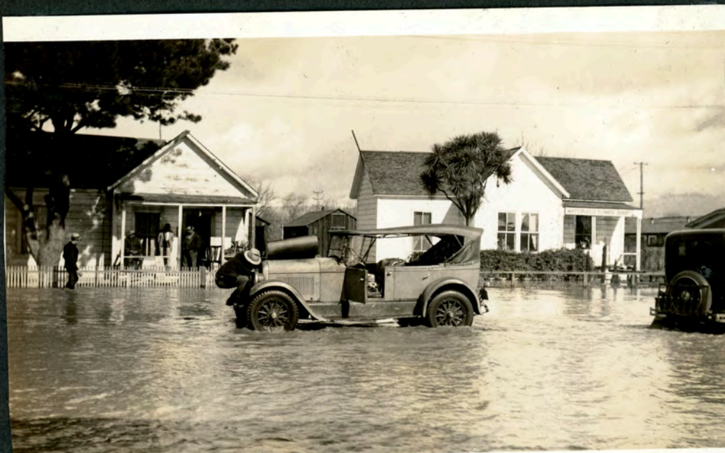
Wet Flood Associated Lane
