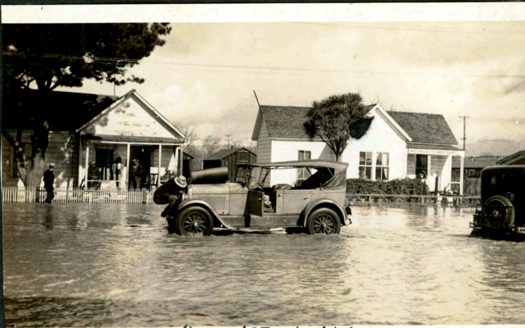
Wet Flood Associated Lane
